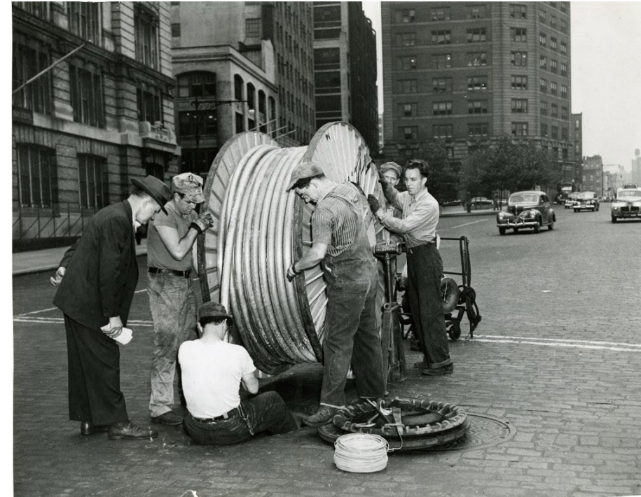
Telephone Cable Being Pulled into Underground Conduit - Lead Covered Cable, Washington, D.C., 1953.
