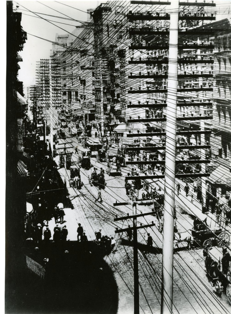
Telephone Pole Line Construction in New York, about 1903
